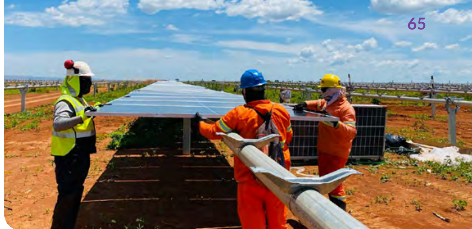
Works on the Janaúba Photovoltaic Solar Complex
