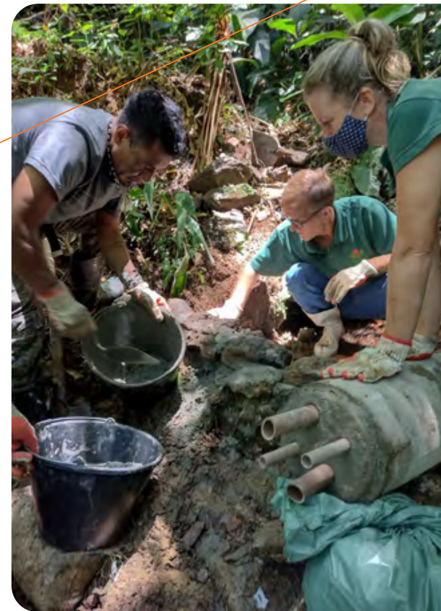
Project Iara - Santa Catarina
