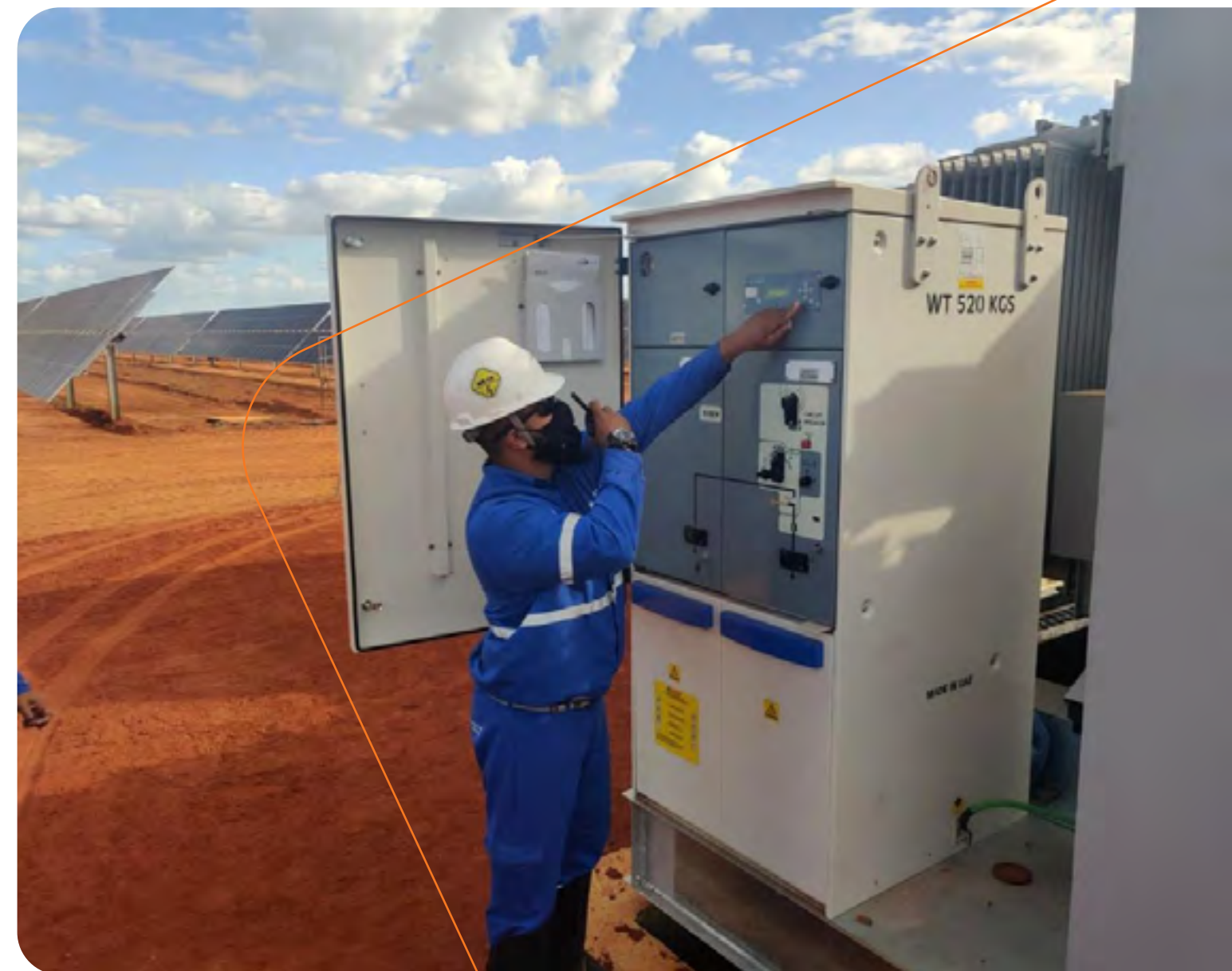
Works on the Alex Photovoltaic Solar Complex
