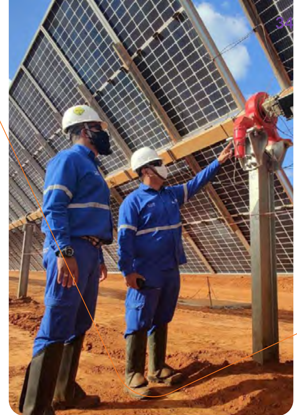
Works on the Alex Photovoltaic Solar Complex
