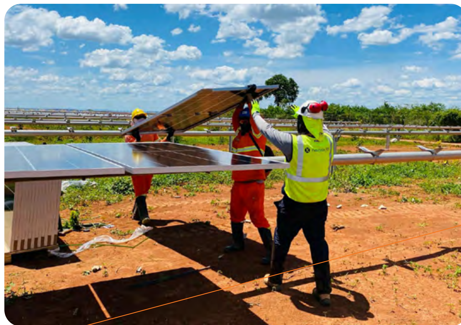
Works on the Janaúba Photovoltaic Solar Complex
